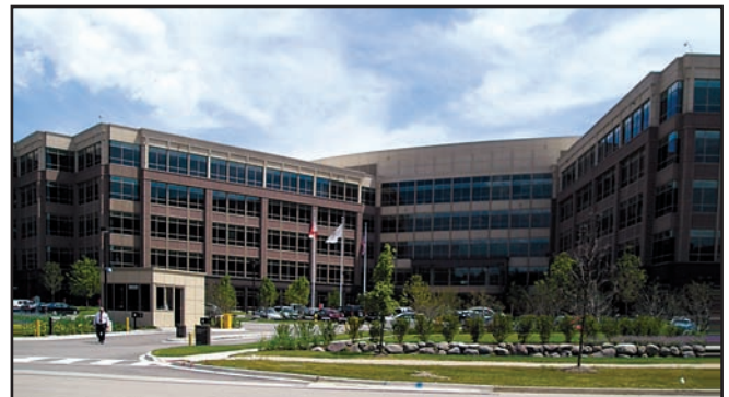
FIGURE 1. The unique shape of the HSBC North American HQ building outside Chicago takes advantage of natural daylight inside the space.
